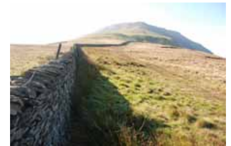
Boundary wall, Simon Fell
