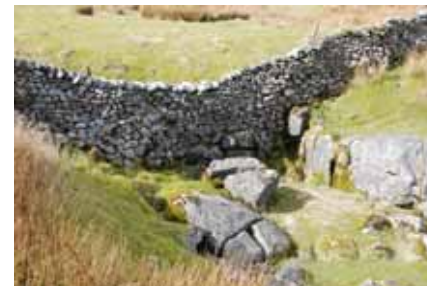
Wall built in dry valley, Ingleborough
